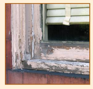
This existing window and its original wooden frame is in poor condition, despite requiring high maintenance for years. Many old wood windows also have issues with dry rot and, in a typical installation of a new replacement window, the dry rot might be covered over with aluminum trim coil rather than replacing the whole window system, providing a larger, darker moist environment in which the fungus will thrive.
